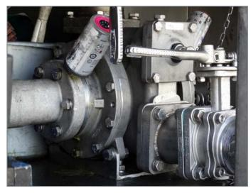
Blackmer® STX Series Sliding Vane Pumps feature a 316 stainless-steel body and internals with chemical-resistant seals, bearings and 0-rings, all of which make it an ideal solution when transferring corrosive liquids like hydrogen peroxide.
